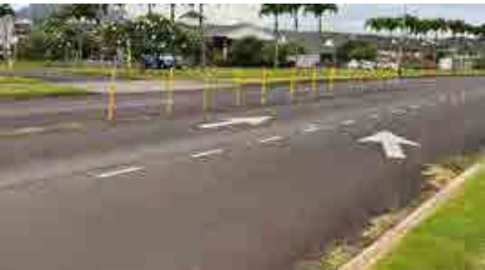
Flexible delineator with rubber curb
